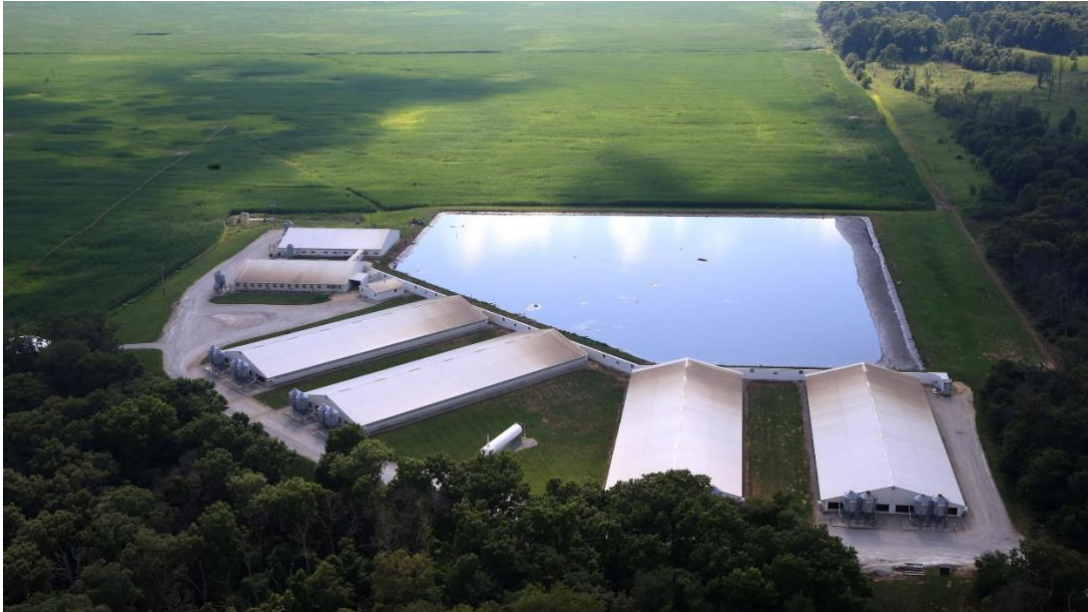
Manure Storage System in Iroquois County, Illinois. 203
